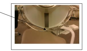
Remove the light deflector. To remove it turn and pull. try not to damage the light bulb.
